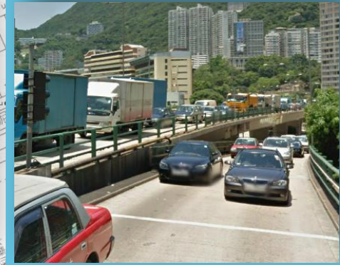
Frequent Weaving Movements at slip road (from Wong Lai Chung and Flyover of Canal Road West) 車輛於橋面支路(由黃泥涌道至堅拿道西天橋)頻密穿插而行
